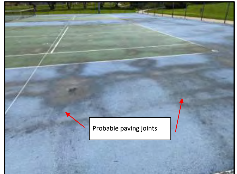
Photo #8 – Low area along paving joints
