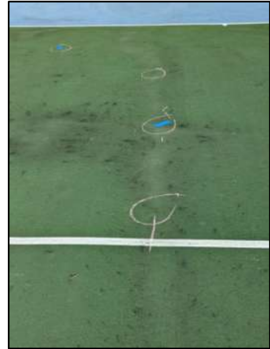
Photo #18 – Settlement over crack
