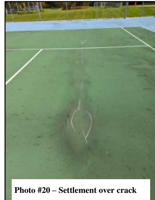
Photo #18 – Settlement over crack
